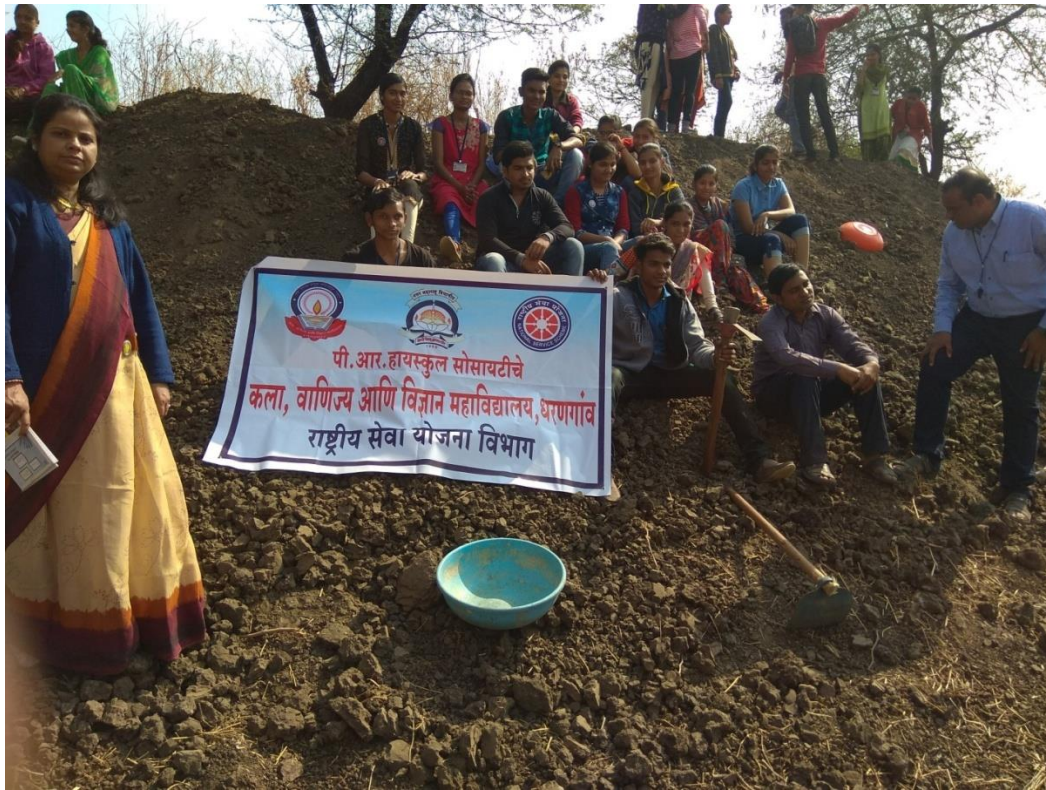
Students Removing Silt From A Dam
